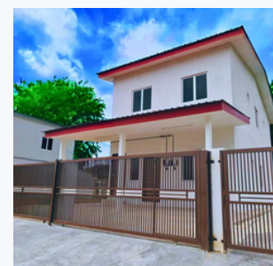
Town house - Fasa 2 (Sg. Merab)
